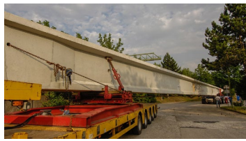
Transportation of overlong concrete parts (up to 50 m and 100 tons)
